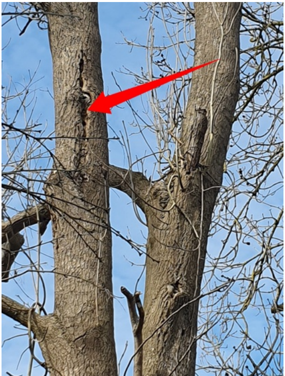
04 P002 Potential decay point
